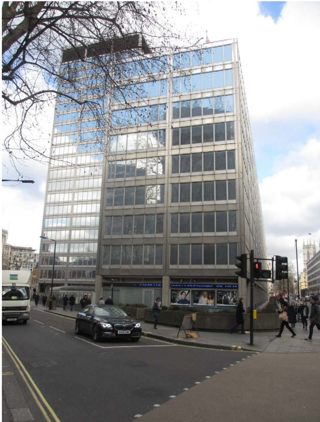
8 – 10 Broadway, New Scotland Yard (view from Victoria Street at corner of Broadway (prior to works))
